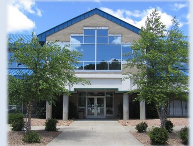
Meticulously Maintained Building and Grounds
