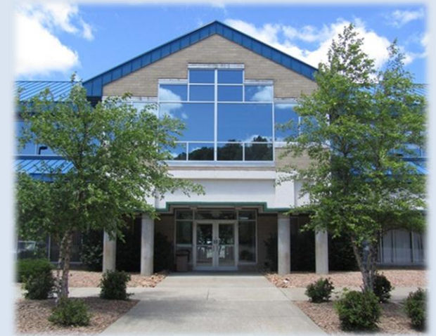
Meticulously Maintained Building and Grounds
